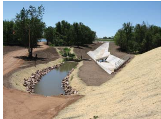
Stubbs & Miller structure and spill channel
